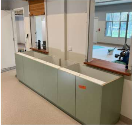
Social Support - joinery installation
