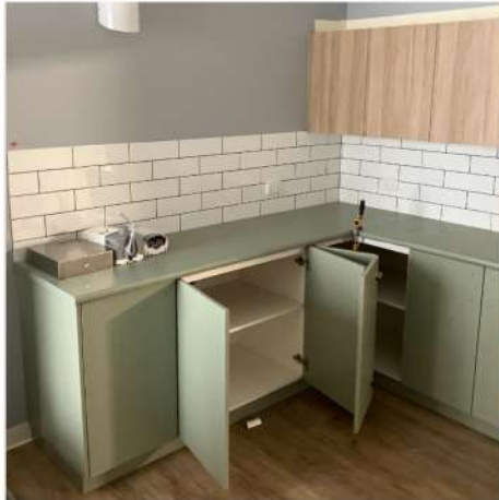
New cabinetry is being fitted
