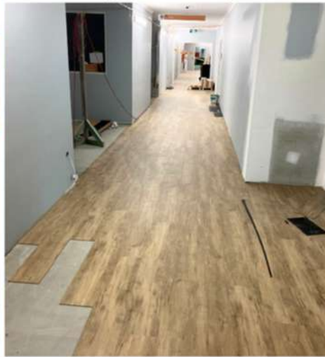
Community Care flooring installation
