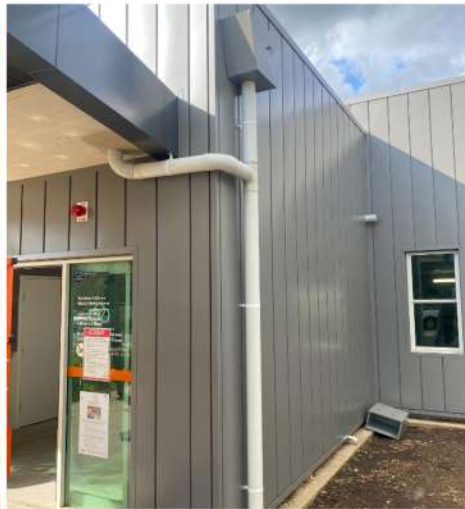
Finishing touches on the cladding
