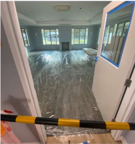
Aged Care Lounge flooring is complete
