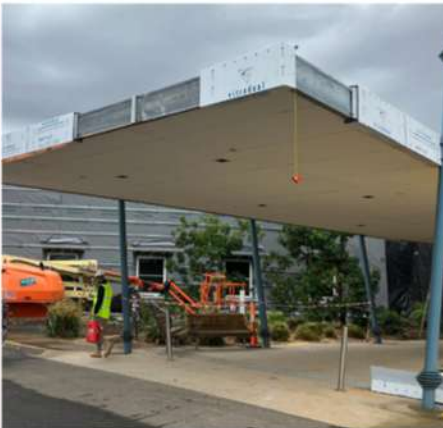
Working on the Main Entrance
