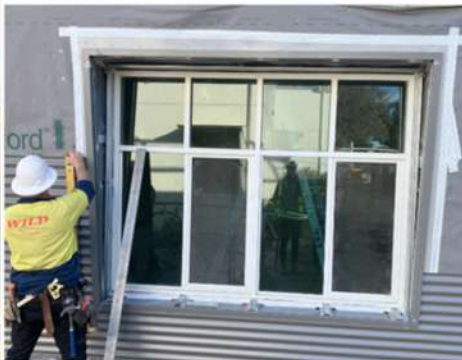
Cladding & window treatment installation
