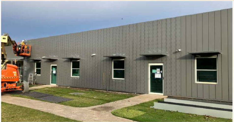
Cladding installation is now underway on the outside of the building
