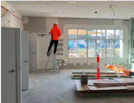
Social Support Room is progressing
