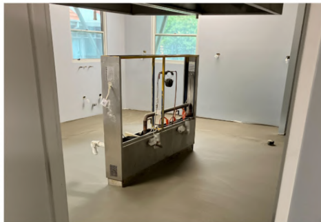
Kitchen refit is progressing
