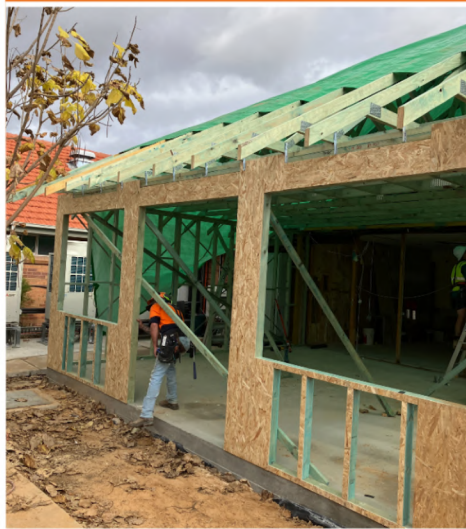
New staff lounge/dining area extension
