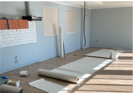
Laying of vinyl in the Acute Care wing
